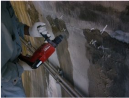
1) Drilling holes in preparation for nipple placement
