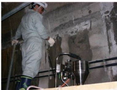
3) High pressure RADCON Formula #7 injection taking place
