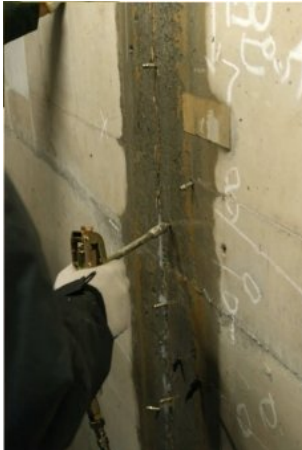
2) Nipples in place, RADCON Formula #7 being injected
