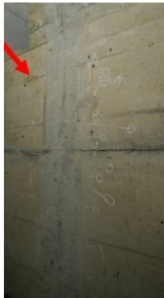
5) Post injection application – a RADCON Formula #7 total lifetime waterproofing solution
